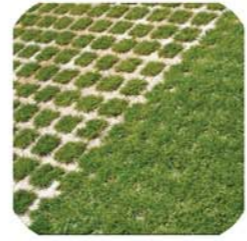
Permeable pavements
