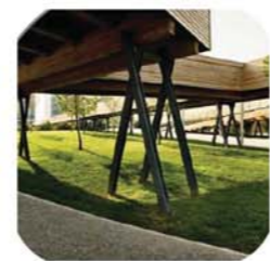
Elevated timber footbridge
